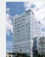
Hachioji ACCT Tower (2001)
